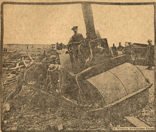
The engineers across the water are constantly busy making roads and reconstructing those that have been torn up by shells. Here is a roller that has got stuck in a ditch, and it takes husky Canadians like those you see to pry it back into place.
