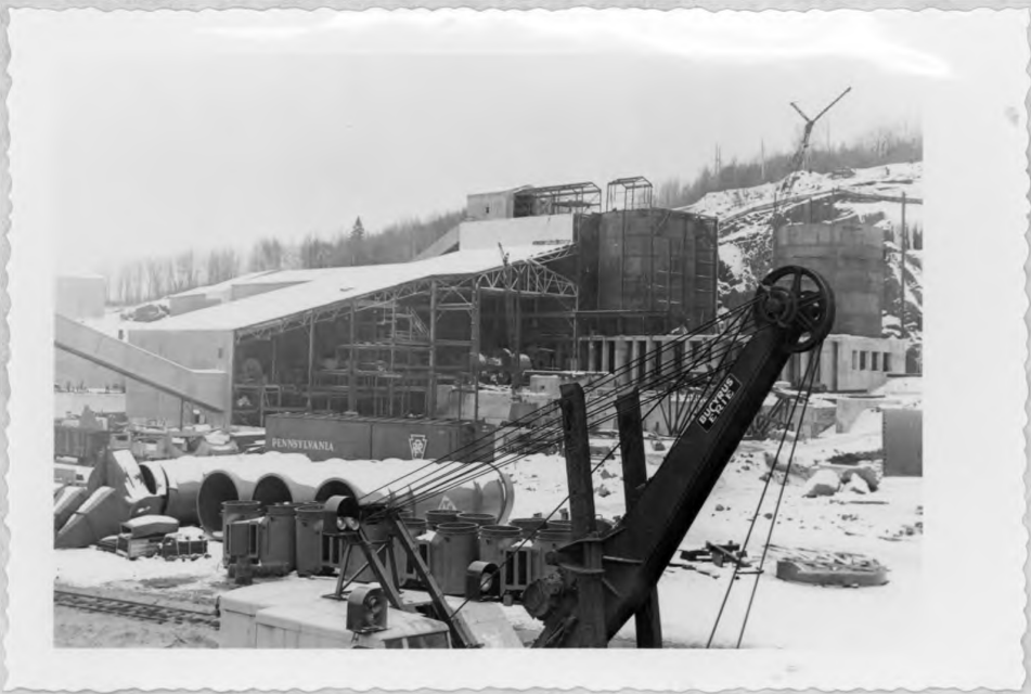
MILL ADDITION LOOKING WEST DECEMBER 1959
