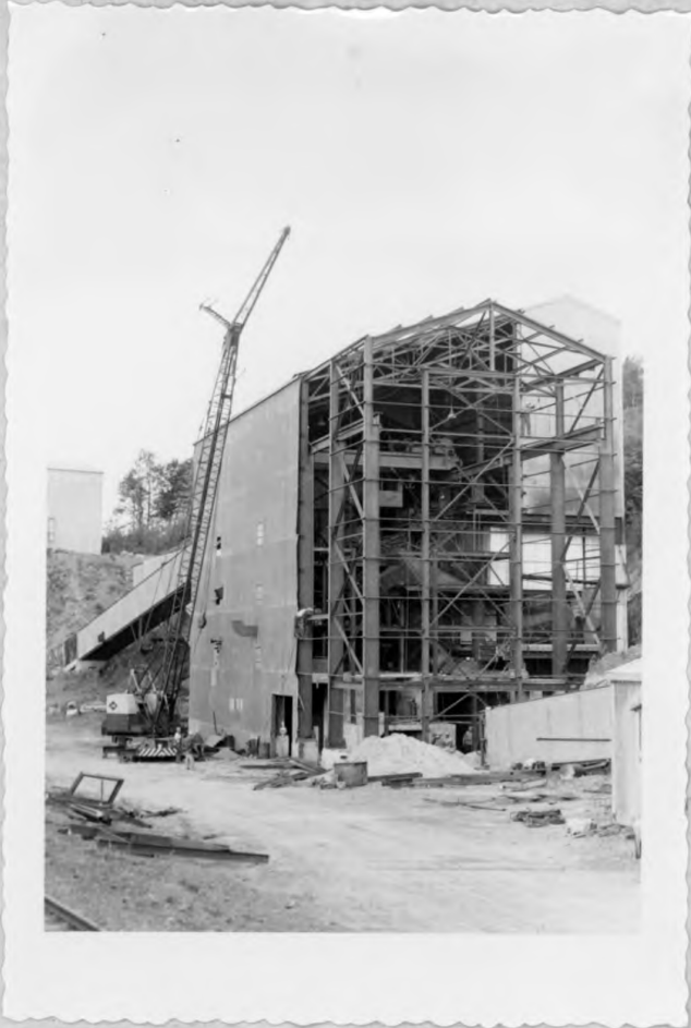
CRUSHING PLANT ADDITION AUGUST 1959
