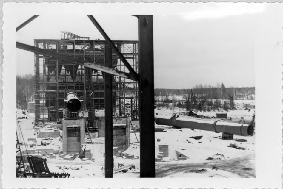
PELLET PLANT - LOOKING EAST DECEMBER 1959
