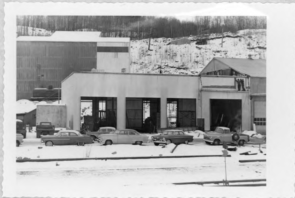
SHOPS ADDITION - DECEMBER 1959
