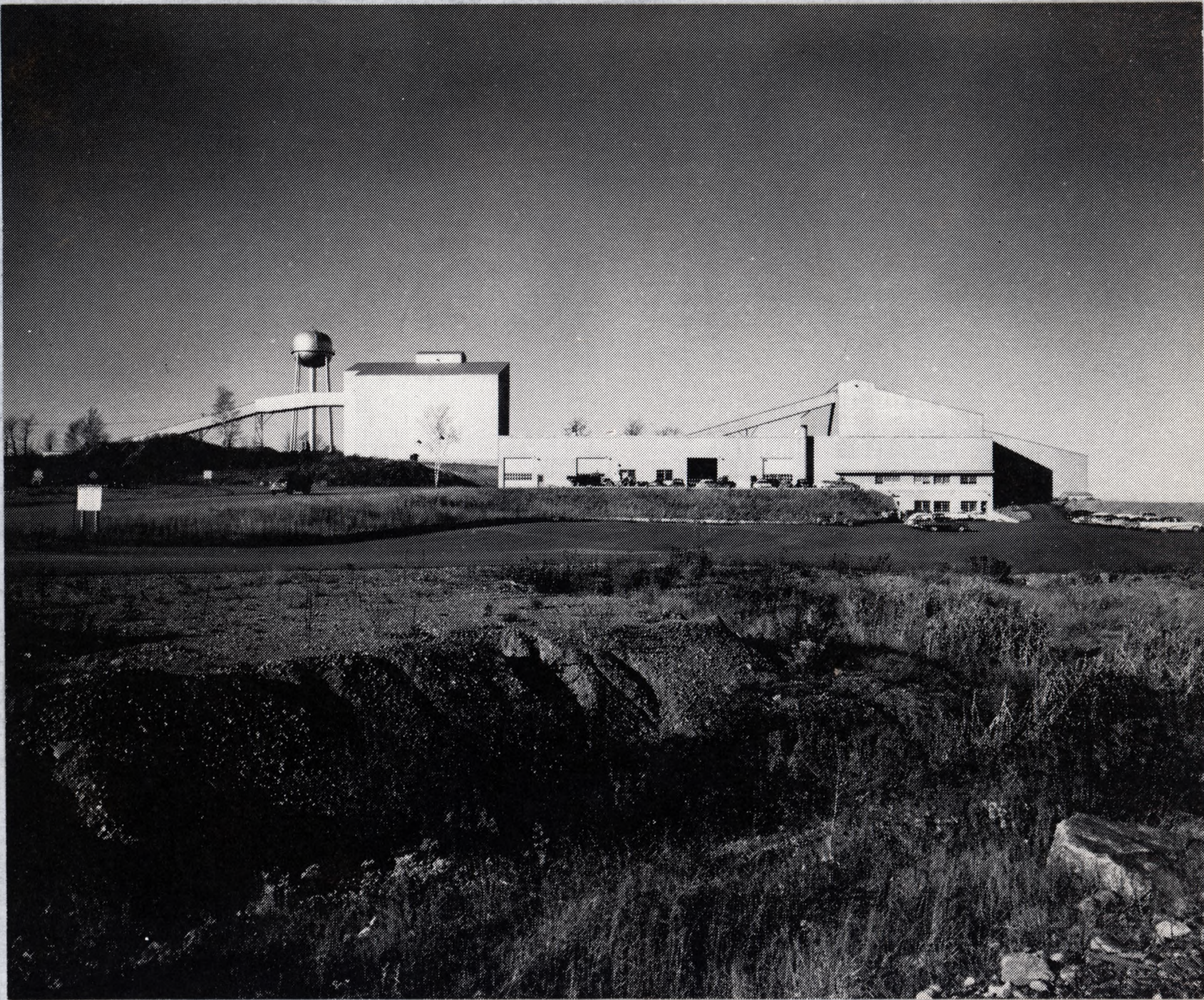
FIG. 1. View looking north, showing secondary-tertiary crusher building on left, shop-office-dry building in foreground and concentrator in background on the right.
