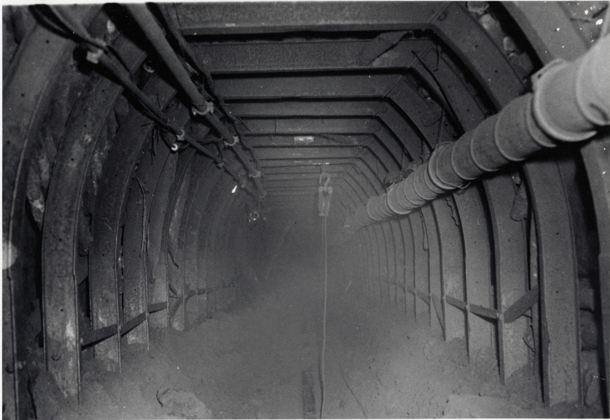
A sub-level conveyor belt drift development using arched legs, which were modified from their original form at the mine shops and straight caps, which also were fabricated at the mine.
