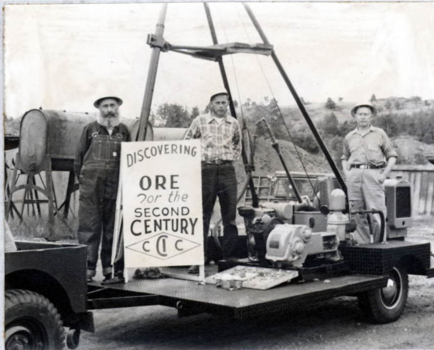
View showing trailer-mounted diamond core drill and pump with tripod mast erected. Picture was taken at the time of the Ishpeming Centennial Parade and includes from left to right, Victor Nelson, Alvin Nelson and Swante Merrila
