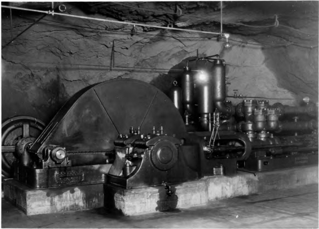
Plate No. 194 Crescott Flunger Pump on 2400 ft. Level Athens Mine
