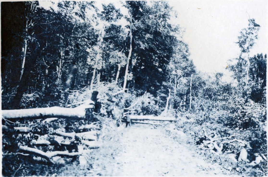
Clearing windfalls from East road after the windstorm.
