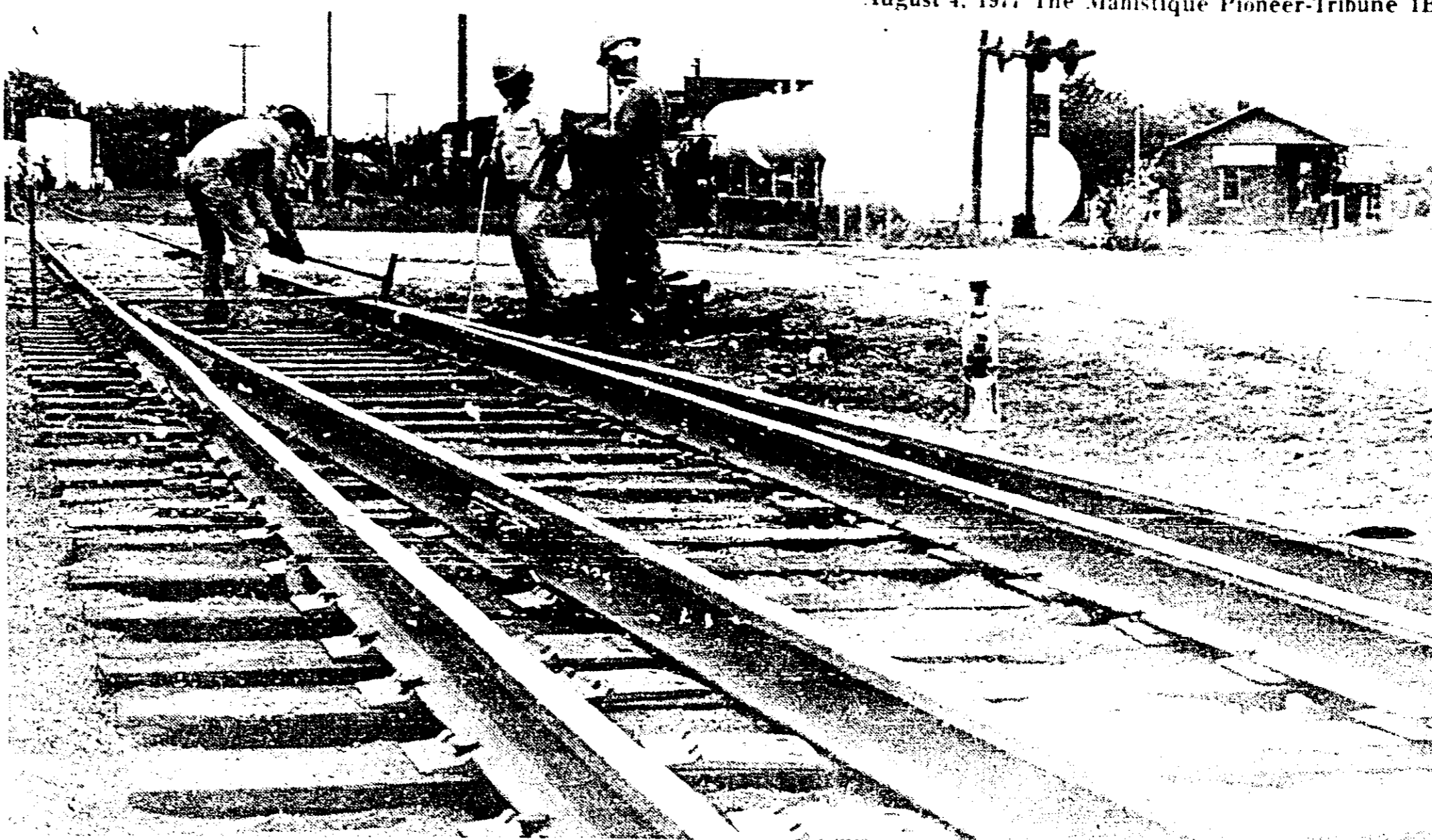
EMPLOYEES OF the Soo Line Railroad have been working this week on installing new tracks and improving the crossing at North Houghton Avenue on Manistique's west side. According to W. J. Howes, roadmaster for Soo Line, one pair of tracks just south of the main running south will be removed. The tracks running south of the station will be joined with the main crossing west of North Houghton. Howes said that will enable them to install gates closer to the main tracks to improve safety conditions in the area. Steve Savoie, left and Paul Drago, both of Manistique; and Rick Keerridge, of Engadine, are shown working on the new tracks. (Tribune photo)
