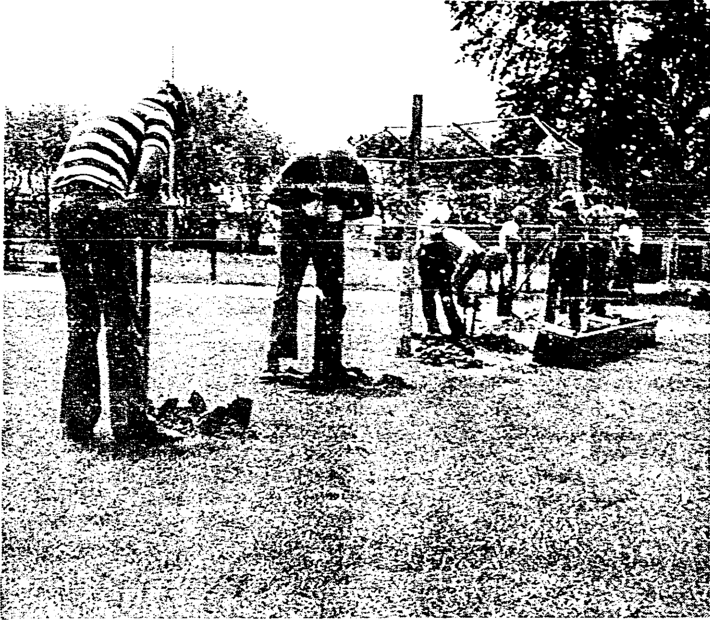
One of four crews currently working under the Youth Conservation Corps, was in Manistee this past week helping Rick Larson, city recreation director, install new fence posts at a ball diamond in Central Field, above photo. The YCC will also help in constructing the Fifth Street Park, currently planned by the city. They should begin work within the next few weeks.
