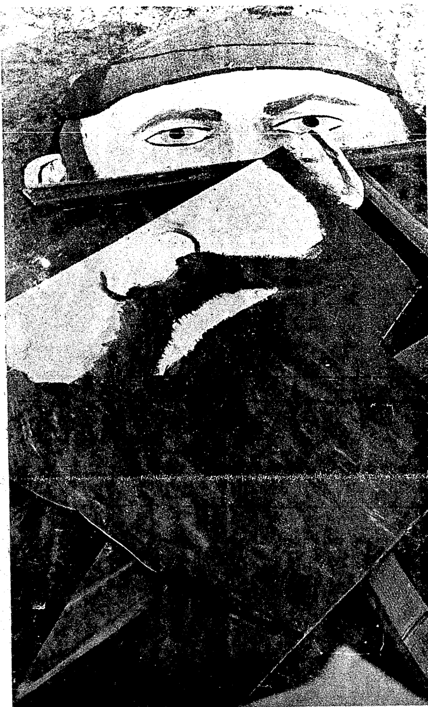
THE CITY'S Paul Bunyan facade lays in shambles after a fierce wind storm
