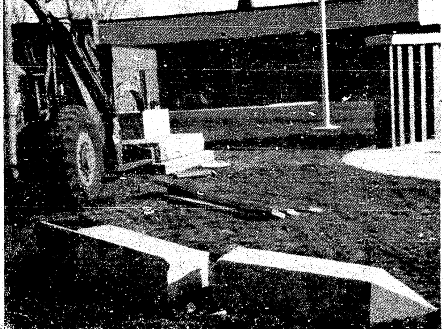
WORLD WAR I monument lay in two pieces Thursday after it toppled off its base as it was being moved by a fork lift tractor. (Photo by F. Clish)
