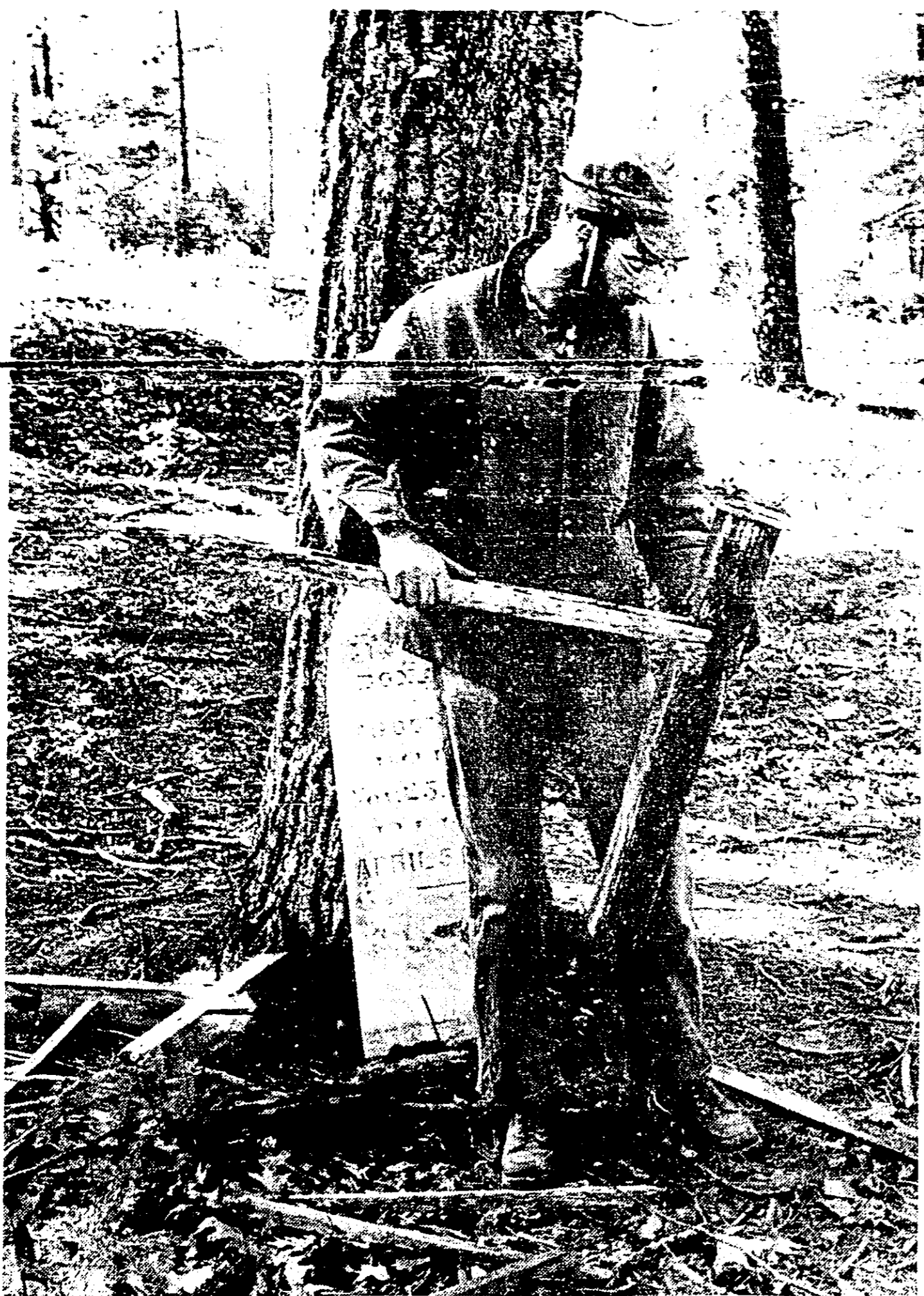
Fayette carpenter, Doug Smith, examines pieces of grave enclosures that will be reconstructed and erected at the site of the cemetery in Fayette. The cemetery is
