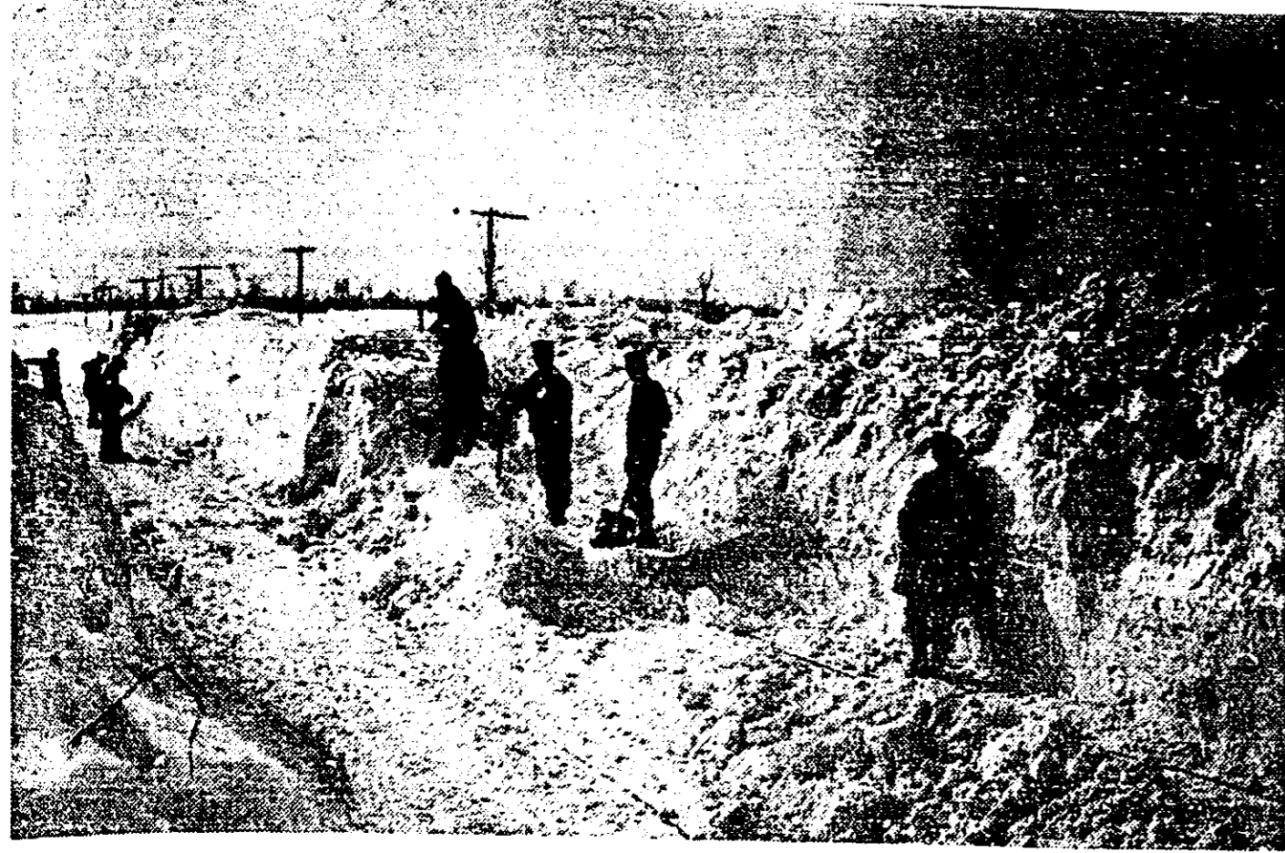
MAX OSTERHOUT of 618 Oak, sent this picture of an early 1900's road crew busily engaged in clearing the road for traffic. The official date of the picture is April 5, 1923. Back then the only way to keep the road open was to have a road crew, each yielding a shovel and a lot of muscle.
