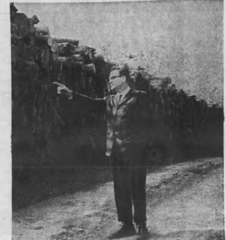
Rep. Mack points to hemlock pulp wood salvage from the right of way of the last five miles of the south boundary road that traverses virgin timber in the Porkies Park. Dry weather during the summer and fall speeded up construction work on the project, which will be completed next year.
