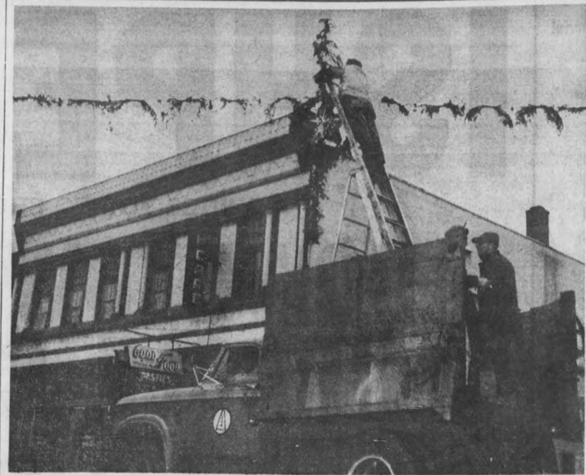
Shown in the process of erecting Christmas decorations in downtown Ishpeming is Les Rock, an employee of the public works department. Over 40 combined wreaths and stars will decorate Ishpeming's intersections.—(Mining Journal photo.)
