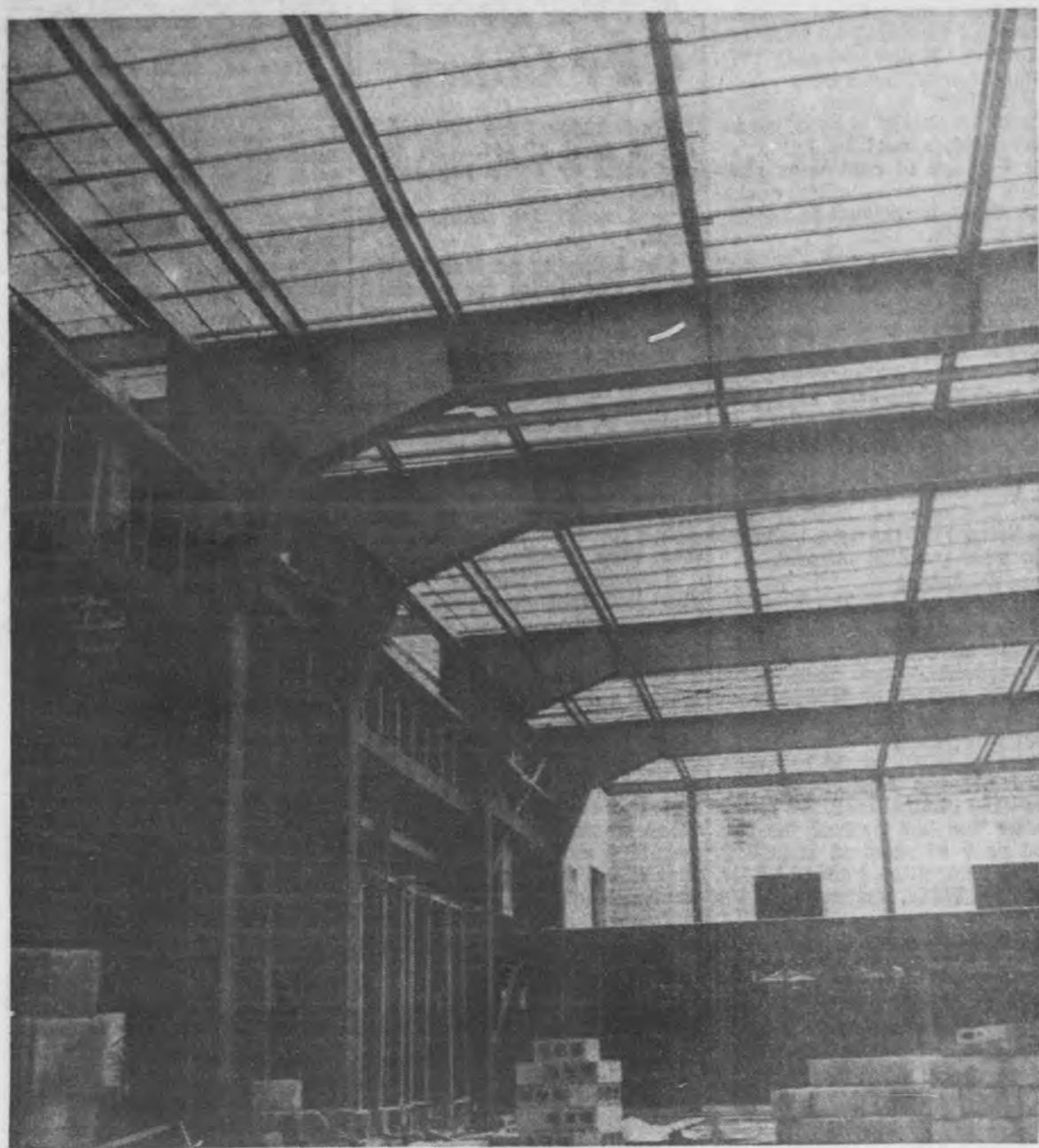
Superstructure for the Marquette Senior High School gymnasium is rapidly nearing completion, as this photo indicates. The gymnasium will provide seating capacity for about 3,000 persons. Work on the high school itself is around half completed. The school will be ready for occupancy next fall. General contractor is Caspian Construction Co. of Caspian. Cost of the entire building will run around $2.5 million. Work began last spring.—(Mining Journal photo.)
