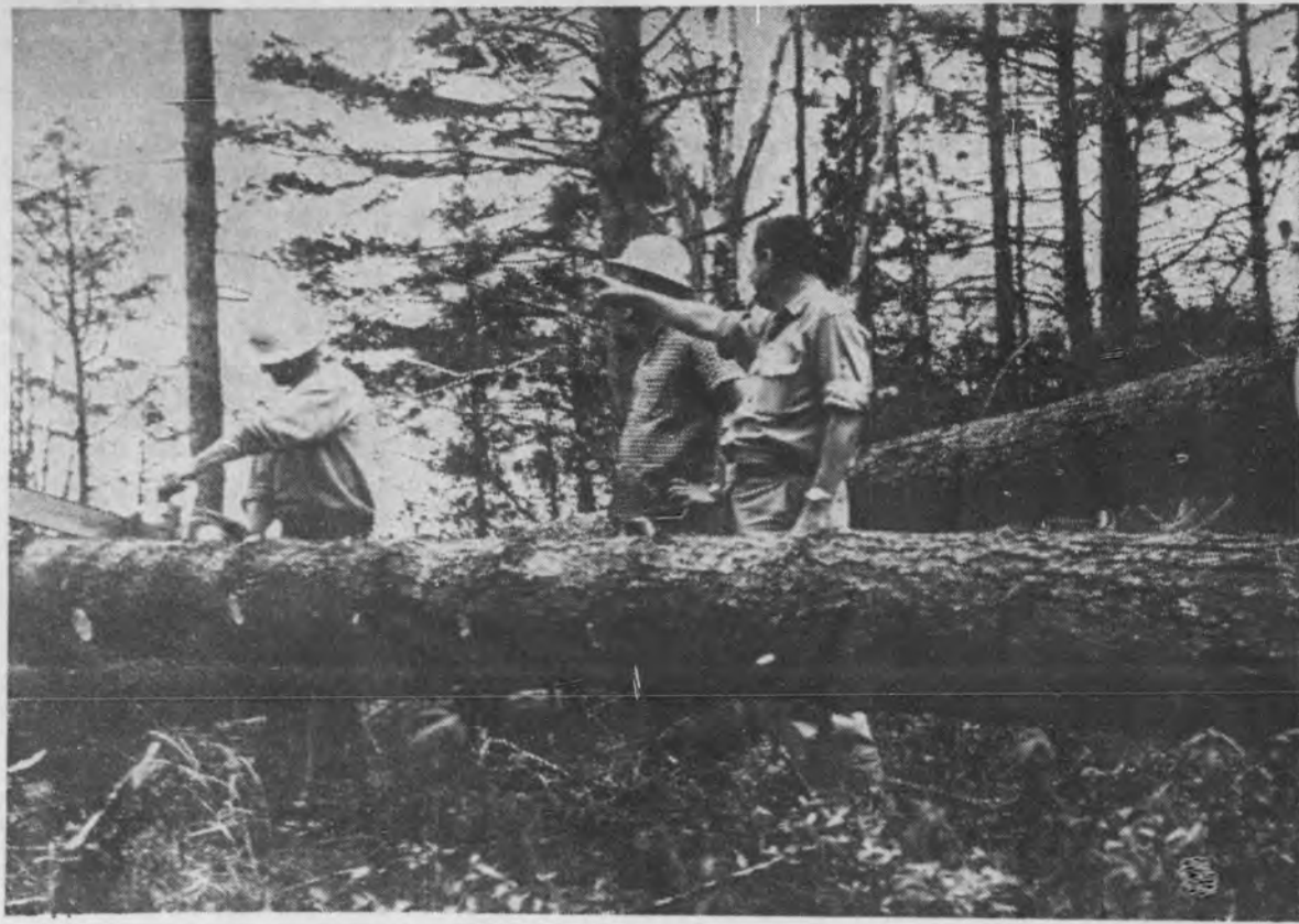
Clarence Forcia of L'Anse begins cutting up felled tree as David Stuck of Manistee, forester and foreman on project, and S. C. Carey, forest manager of Bureau of Indian Affairs, discuss which trees should be removed for new road across swamp leading to beach, where campground and trailer park is under construction north of Baraga.
