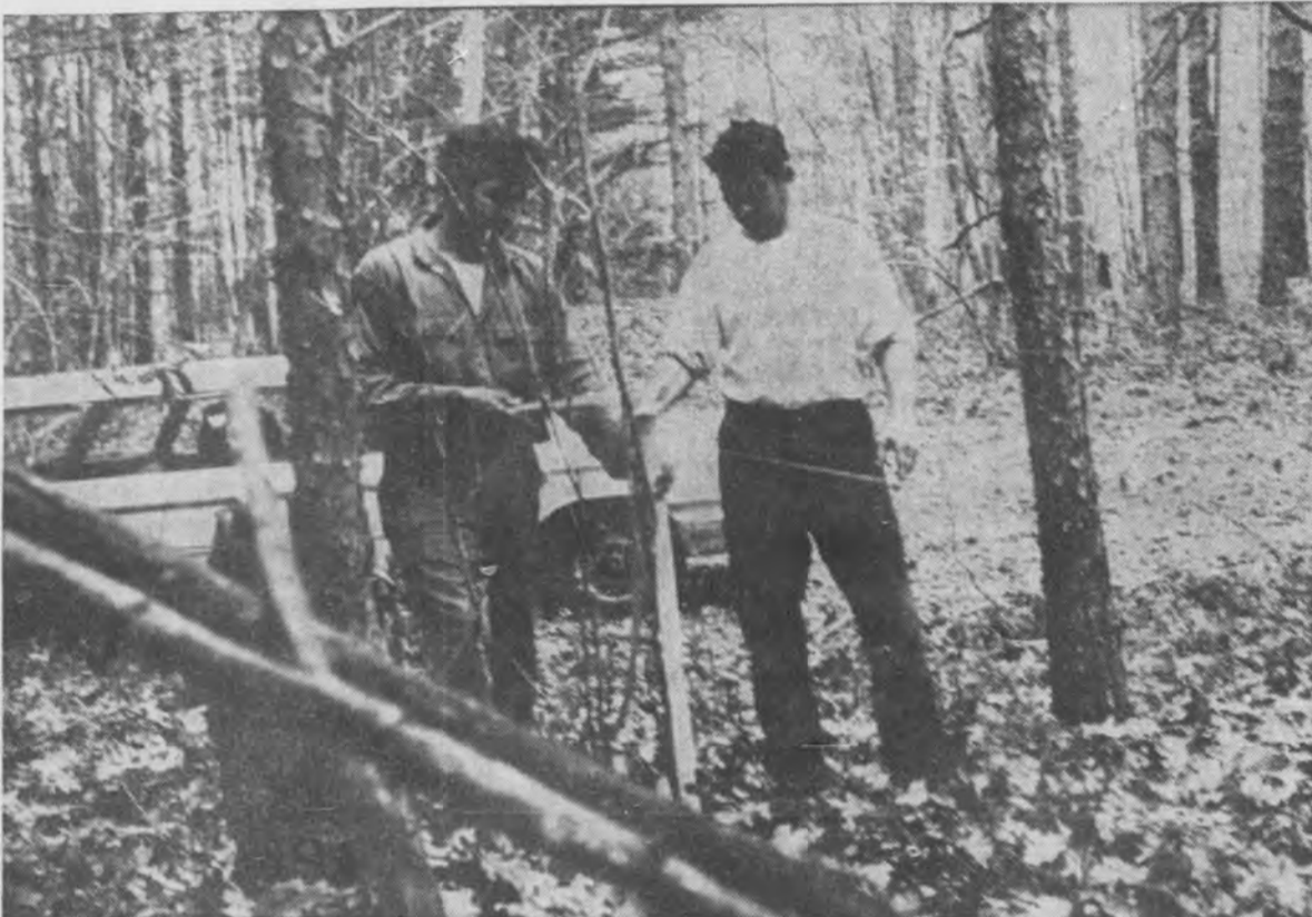
Frederick Gauthier and Hubert Morin, employed on campground and trailer park project being constructed on Keweenaw Bay Chippewa Indian lands north of Baraga, stake out trailer
