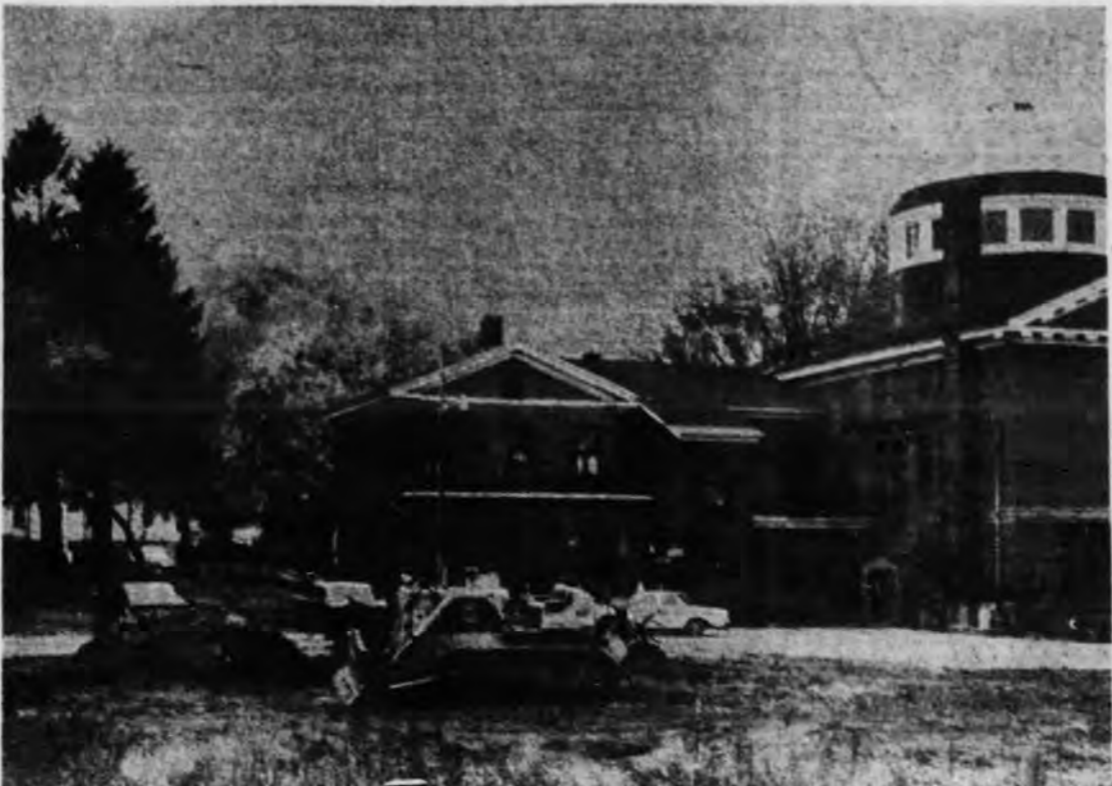
Ground is shown being cleared in Munising, erected on the southeast corner of the court for construction of a new county jail, to be house property.—(Hallifax photo).
