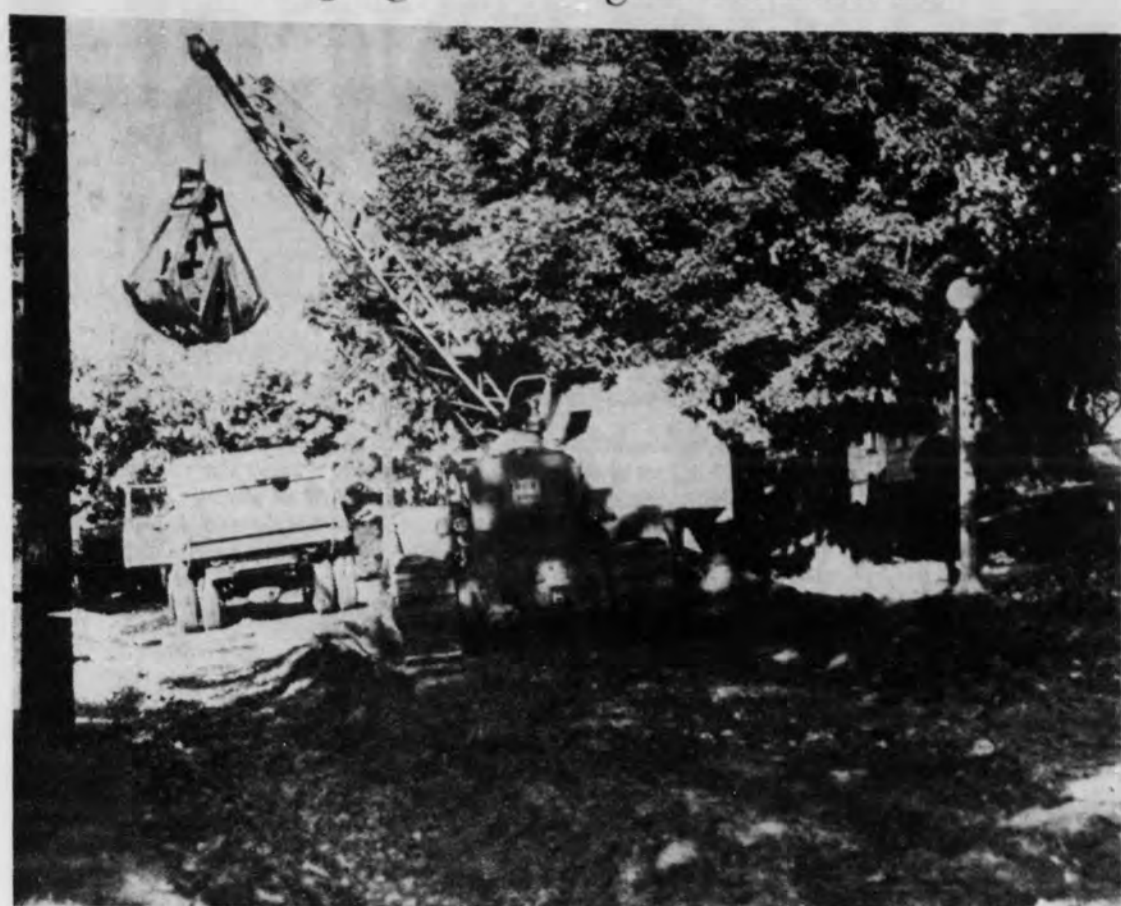
Public works department crews this week began to reshape the pavement on W. Bluff St., west of Fifth St. An excess crown in the street made parking difficult, especially during the winter, and residents petitioned for its removal. The reshaping work also will make snowplow-
