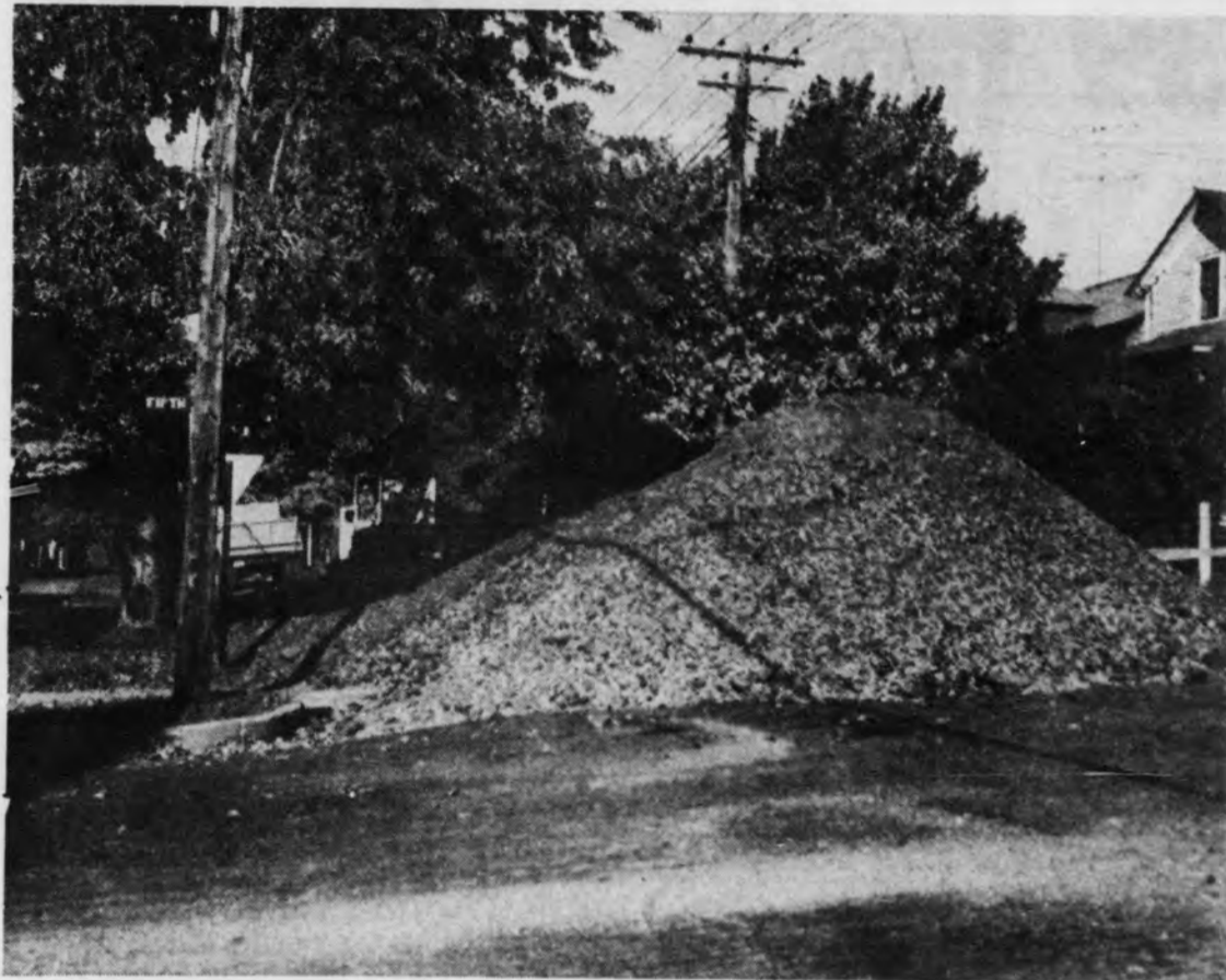
Public works department crews this week began to reshape the pavement on W. Bluff St., west of Fifth St. An excess crown in the street made parking difficult, especially during the winter, and residents petitioned for its removal. The reshaping work also will make snowplow-
