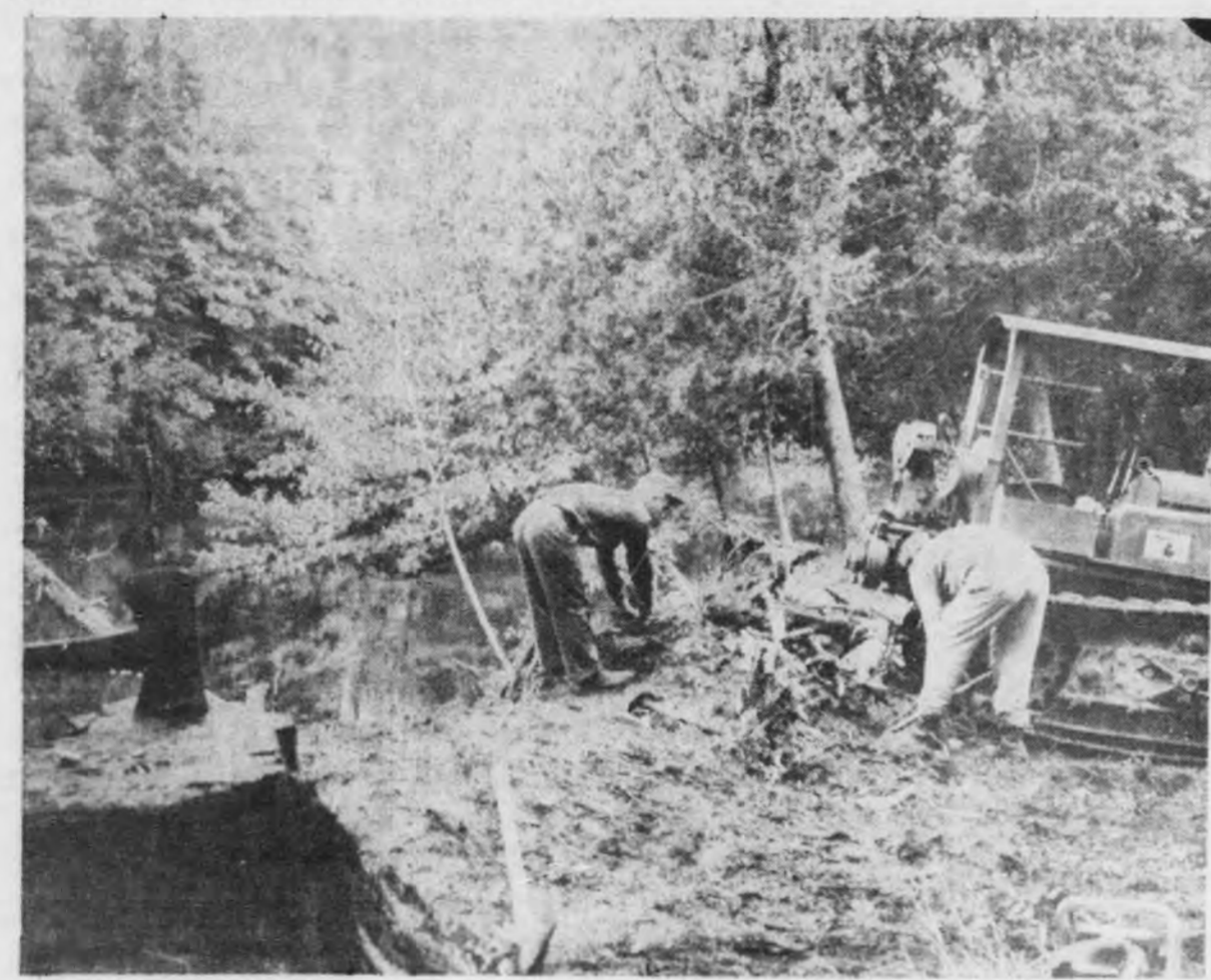
Two local laborers are shown above brushing and burning while bulldozer in background rips out stump near river's edge, where boat launching ramp will be located for public fishing site on Silver River north of L'Anse. Lower photo shows
