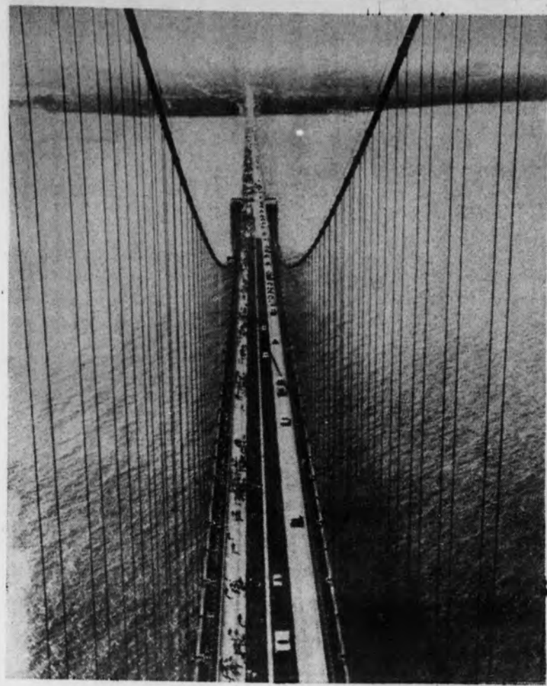
A portion of the crowd of 4,000 people who walked across the Mackinac Bridge on Labor Day in 1962. The Mackinac Bridge Authority expects up to 6,000 people for the sixth annual open recreational walk across the bridge starting at the south end at 10 a. m. Sept. 2. Free transportation is furnished back to the starting line.
