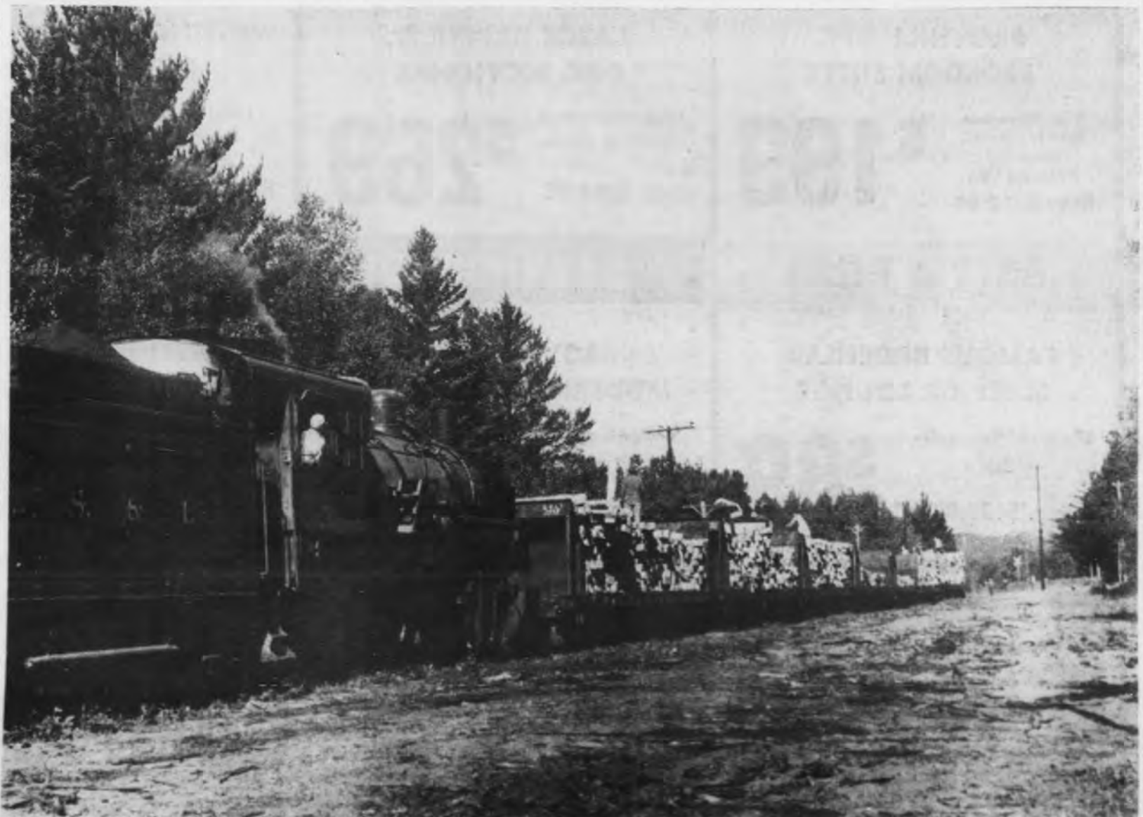
An old LS&I steam engine, now part of the Superiorland project, came out of retirement last week to take part in rehabilitation of the railroad track from Marquette to Big Bay. Here crews dump railroad ties for repair of the line, which had not been used since 1959. Coal tender can be seen at left.
