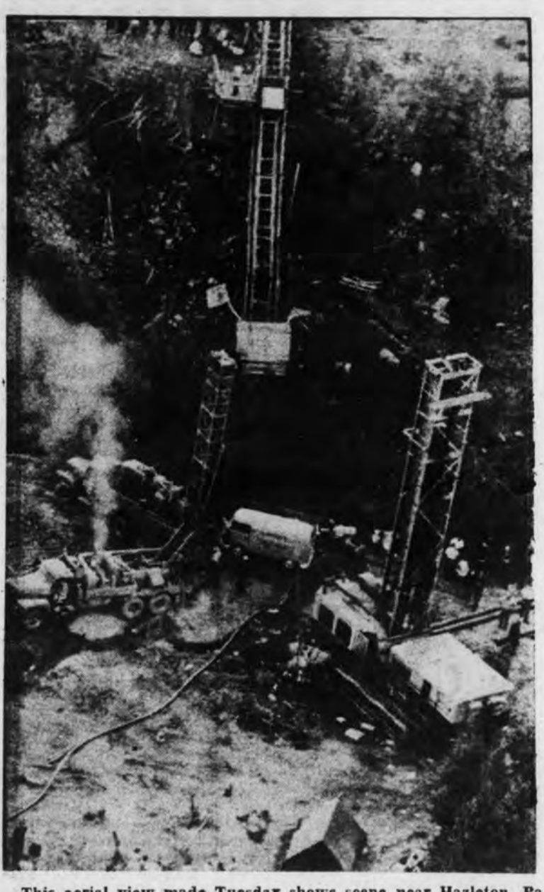
This aerial view made Tuesday shows scene near Hazleton, Pa., where rescue workers are trying to reach three coal miners who have been trapped underground since Aug. 13. At top is railway leading to entrance to mine shaft near center of photo. Big drill driving 12-inch access hole to miners is at right. Rig driving six-inch hole toward third injured miner is at left. Tent for workers is in foreground.
