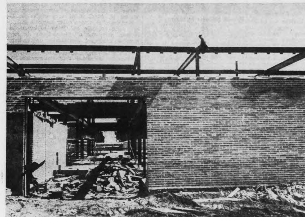
Framework and brick for the new Marquette Senior High School are rapidly going up at the construction site in the Piqua Location. Upper photo shows the steelwork for southwest corner of the second floor classroom. Lower picture is of the outside kitchen wall and of the doorway leading to the receiving and boiler rooms. Caspian Construction Co. of Caspian has the general construction contract. Work began last spring and construction is scheduled to be completed by the fall of 1964. Caspian Construction's general contract is for $1,544,000. Separate contracts were let for the electrical and mechanical projects. — (Joe Sullivan photos.)
