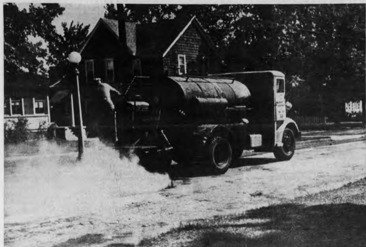
City crews and equipment are shown being used in the city's seal coating program. Above, Clarence Dobbs, tank operator for the public works department, handles the spreader on the asphalt tanker (which is owned by the city) while work is being done on Waldo St., near the Northern Michigan University campus. Below, the pea gravel is dropped into the hot asphalt by the chip spreader, which follows the tanker in the seal coating
