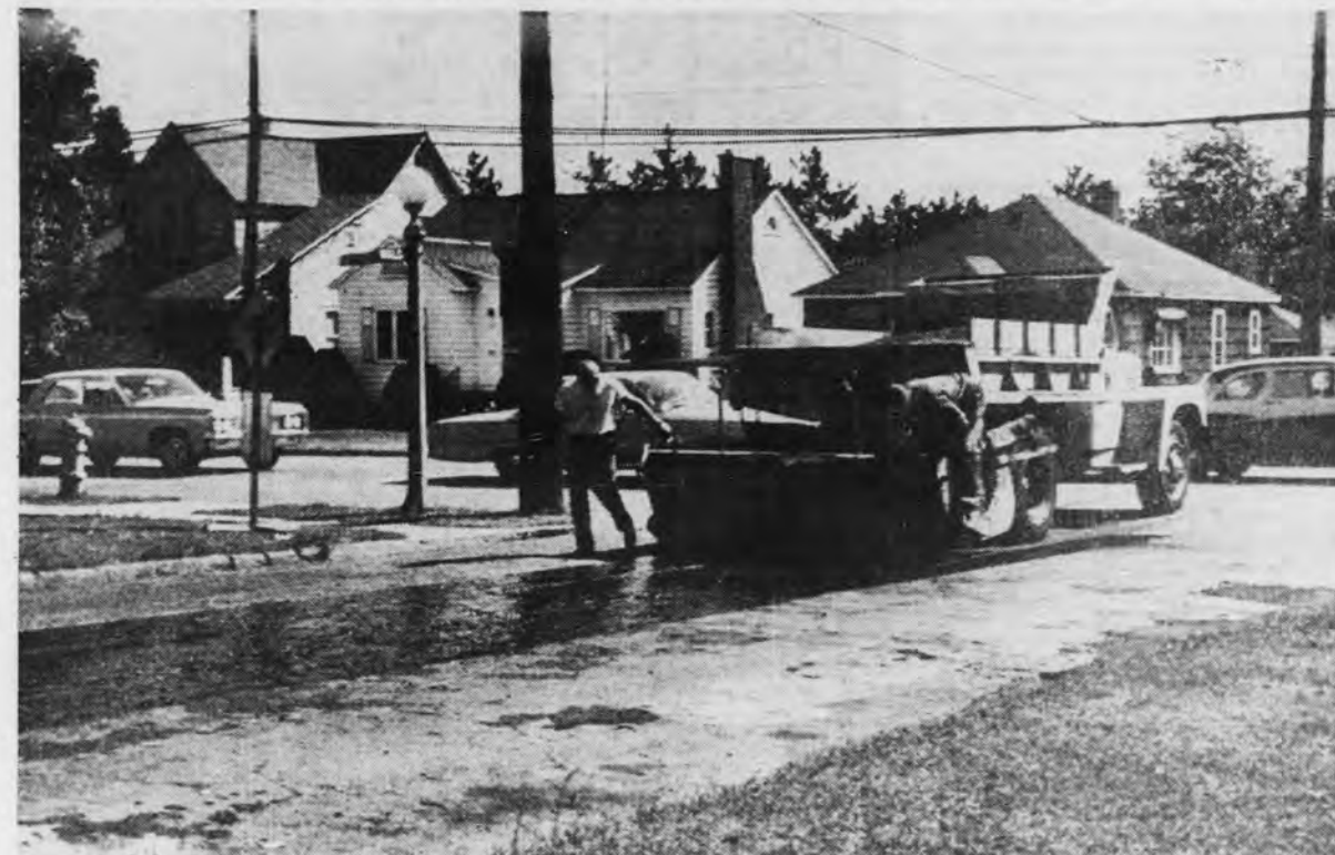
City crews and equipment are shown being used in the city's seal coating program. Above, Clarence Dobbs, tank operator for the public works department, handles the spreader on the asphalt tanker (which is owned by the city) while work is being done on Waldo St., near the Northern Michigan University campus. Below, the pea gravel is dropped into the hot asphalt by the chip spreader, which follows the tanker in the seal coating
