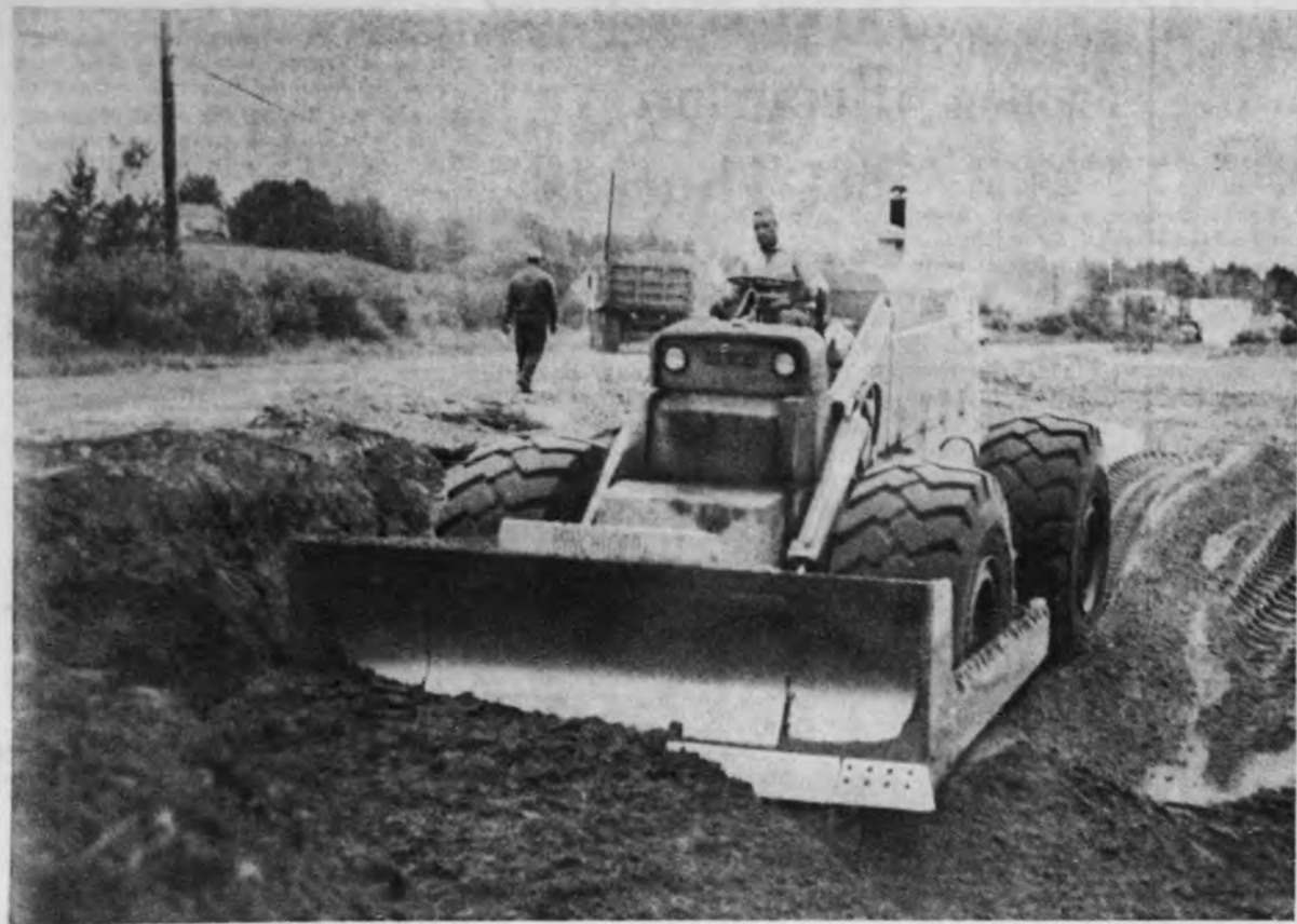
The M-28 business route in West Ishpeming, Mich. has always been in bad shape because of the poor base on which it was originally built, is now being improved. These photos show crews of A. Lindberg & Sons, Ishpeming general contractors, at work on the new roadway. In top photo a huge Michigan-280 heavy duty bulldozer is engaged in backfilling. (Mining Journal photos.)
