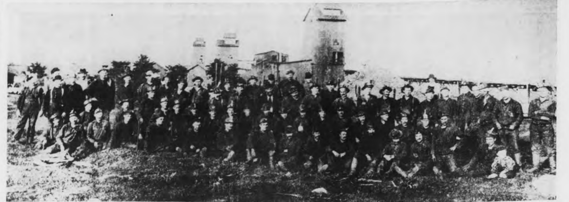
This picture of a group of 19th century miners pictured from left to right are No. 4, 5 and 6, Shaft No. No. 7, is off to the right of this picture. Iron ore has been taken at the Champion Mine in the 1890's. Shaft houses 4 caved in on New Year's Day, 1900. The present shaft, mined at Champion since 1863.
