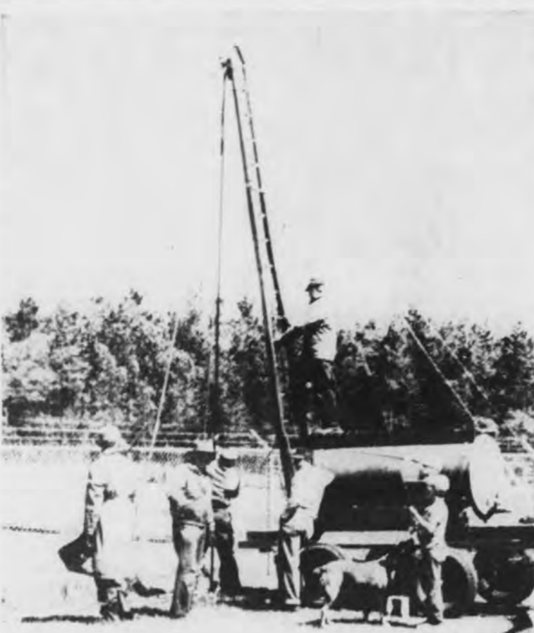
Conservation department crews drive point for one of 10 wells that will supply ground water for lake trout hatching operations at Marquette Fish Hatchery. (Mining Journal photo.)
