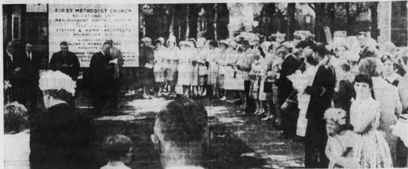
Part of the First Methodist congregation attending the noon ground-breaking ceremonies Sunday in connection with the building of a new educational unit at the church were caught in this photo by James Gooch. The new structure, to be built at a cost of $225,000, will face on E. Ridge St. and will occupy a site where two residences owned by the church were recently torn down.
