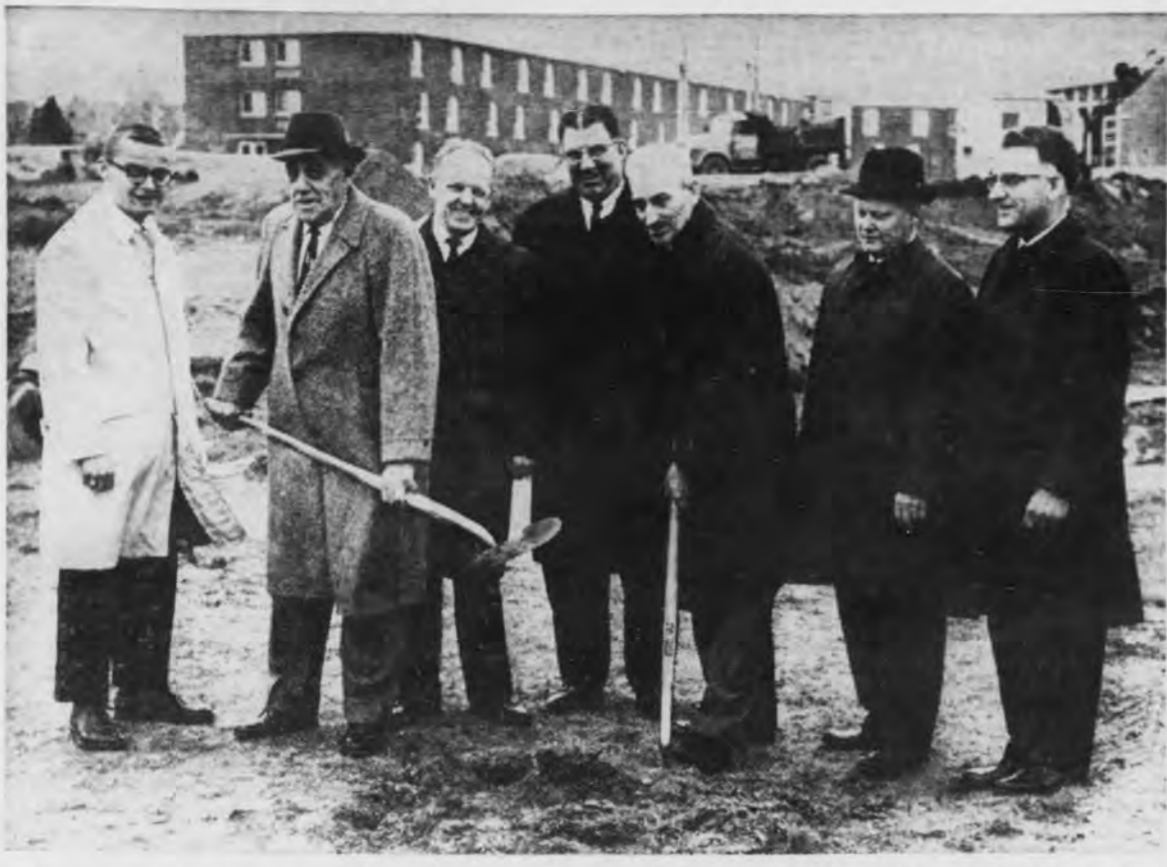
Ground was broken yesterday for the one million dollar addition to the University Center of Northern Michigan University in its east campus. The building, which will be linked to the existing University Center, is scheduled for completion in January 1964. Miller, Davis and Macdonald Co. of Kalamazoo and Marquette has the general contract for the project. Shown at the ground breaking are, from left, James Surrall, Newberry senior president of the NMU Student Council; City Commissioner Steve A. E. Johnson; Dr. Allan L. Niemi, NMU dean of students; Dr. Edgar L. Harden, president of NMU; City Commissioner Joseph Fine; Harlan Larson, president, Marquette Chamber of Commerce; and Dr. Claud A. Rosworth, vice president for public services, NMU.—(Mining Journal photo).
