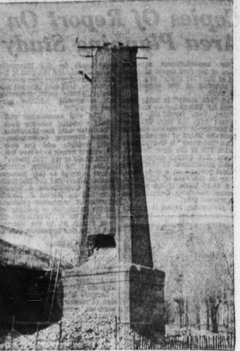
Signs of the times at Northern Michigan College show an old chimney coming down. The unused smokestack, a landmark for more than 50 years, became obsolete when new, larger heating plant was built. Steeplejacks with crowbars reduced the 125-foot stack to a small pile of bricks in a few days.—(NMC photos).
