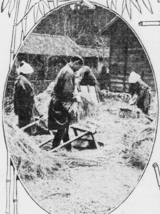
STRIPPING OFF THE RICE GRAINS BY DRAWING STALK THROUGH TOOTHED FRAMES
