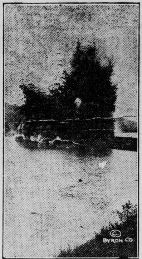
Blowing Up of Gamboa Dike.
