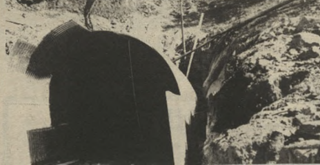
The tunnel of gold, Ropes Mine, is northwest of Ishpeming. It will produce about 30,000 ounces of gold a year when in full operation. (Photos by David Schneider)
