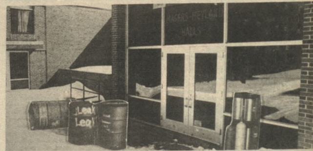
Magers and Meyland Halls have already become the storage site for chemical wastes. Officials say
