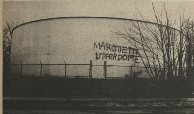
In a city where it can snow over "spring" break, and have hurricane strength winds from three different directions at once nothing seems impossible. Nothing, that is, except this storage tank which
