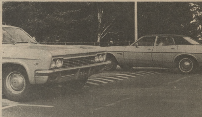
According to Ernest Neumann, all speed bumps may be extended across the entire road width (as above) in order to prevent drivers from swerving around them.
