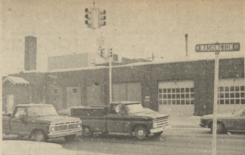
AFTER YEARS OF RED TAPE and waiting, Marquette became the proud mother of two fully operating alternate blinking 4 traffic lights. The lights were installed at the corner of Washington and Lincoln to alleviate congestion during rush hour. (Rush hour is from 4 p.m. to 4:10 p.m. on Thursdays. Catch it some week as an alternative to watching the fruit trucks unload at Anglies.)
