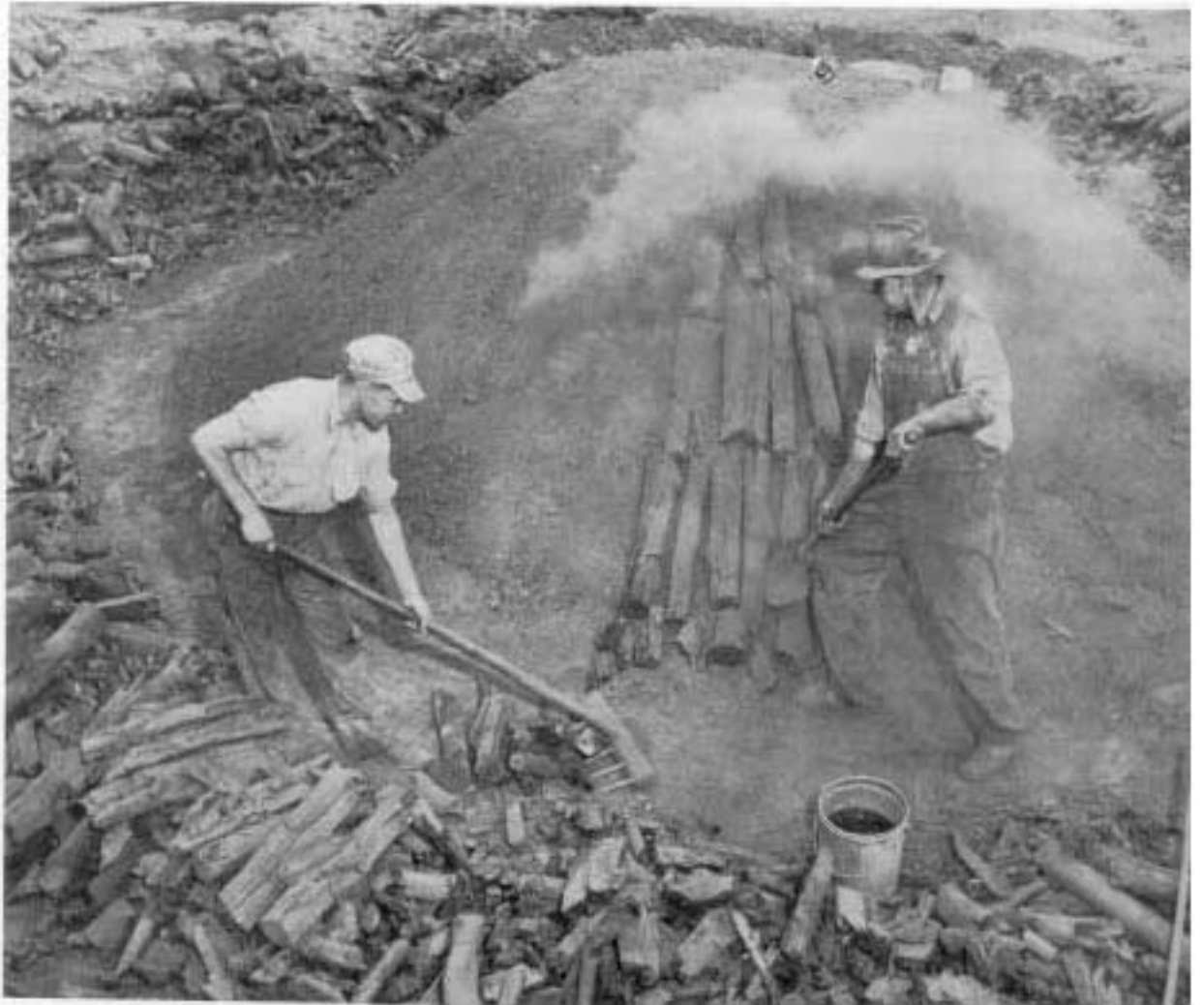
Figure 1. --Early charcoal production in earth kilns.
