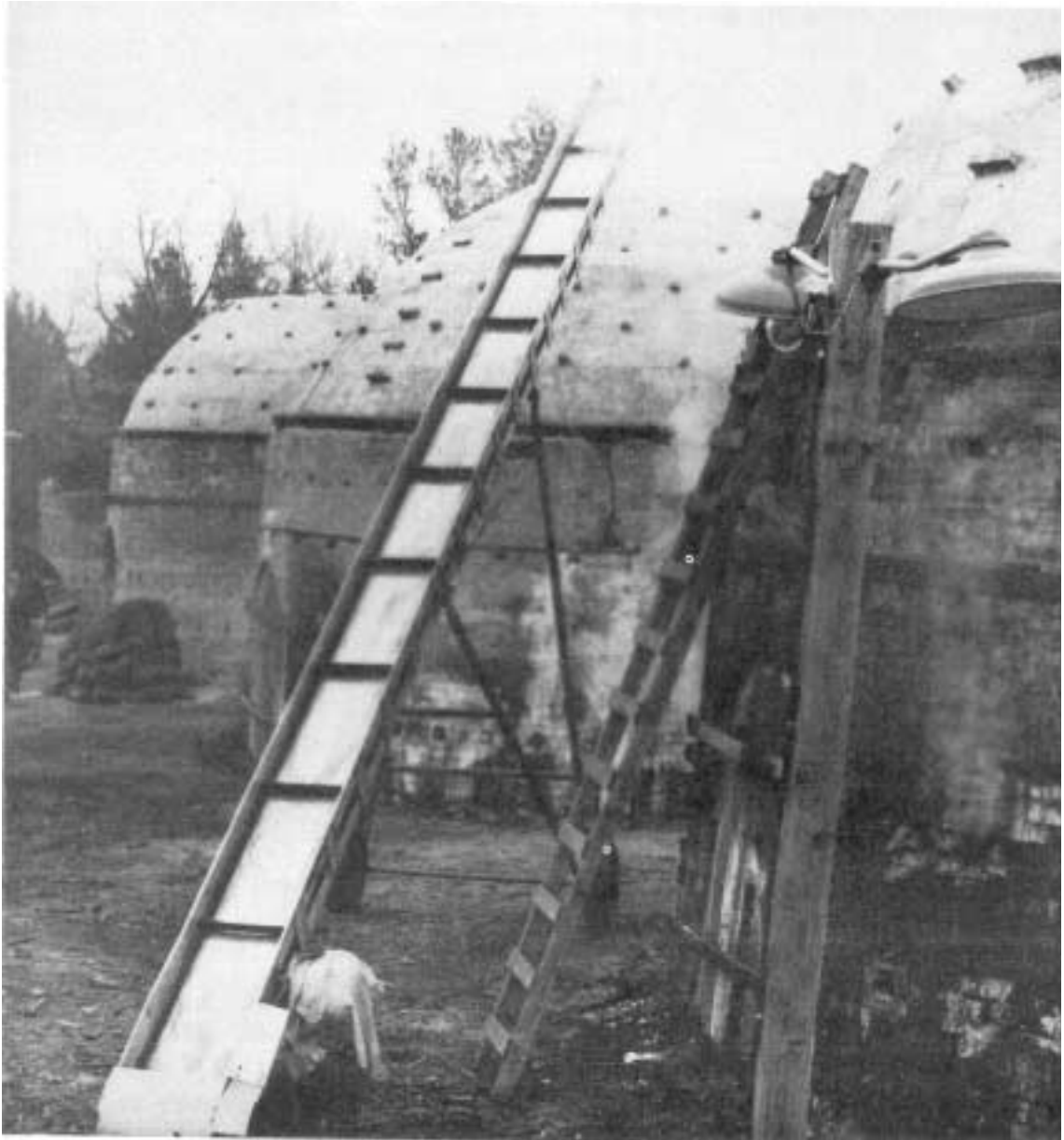
Figure 3. - -Beehive kilns - - recent construction of 75-cord units.
