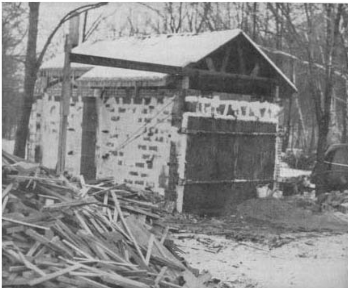
Figure 15. --Experimental single-wall, masonry block kiln.
