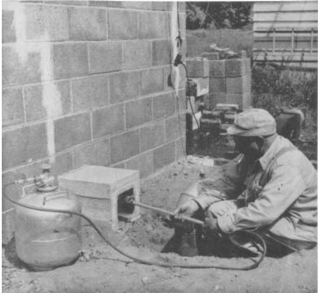
Figure 31. - - Igniting the kiln charge with a torch.
