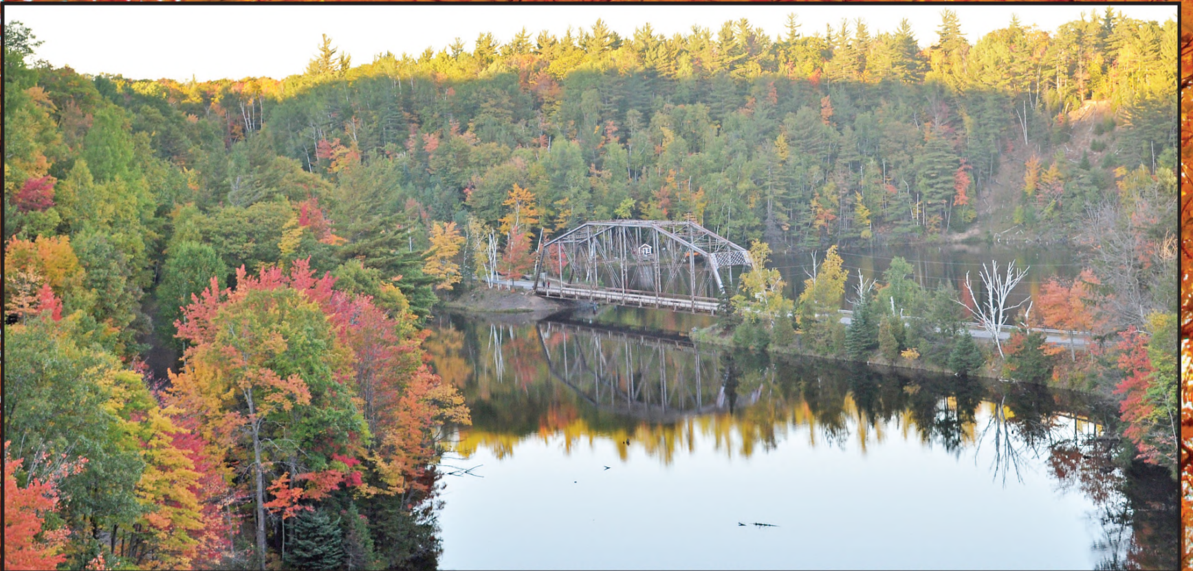
Above: The old bridge located off of County Road 510. With the peak of the fall colors coming up soon, be sure to get a hike in before the snow hits.
