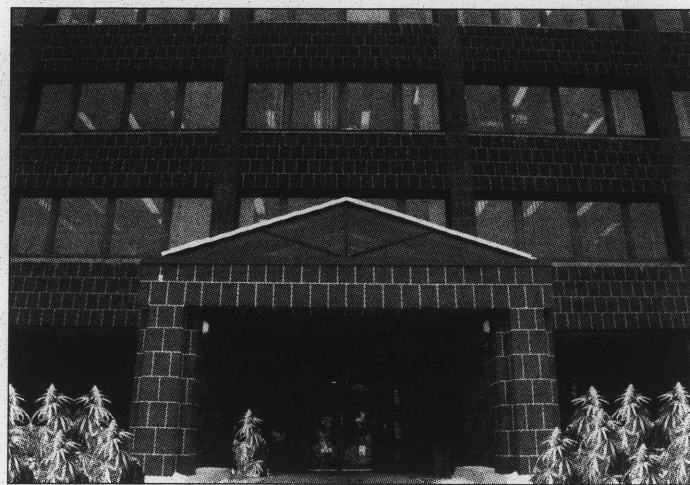
Photo illustration by Manbe Pettin-Kitties/SB NMU administrators have been throwing seeds out of windows, causing a jungle of marijuana plants to grow around Cohmonus.
