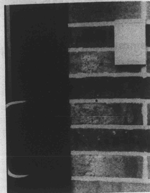
New key card system saves energy while monitoring doors. (Guy Keplinger photo)
