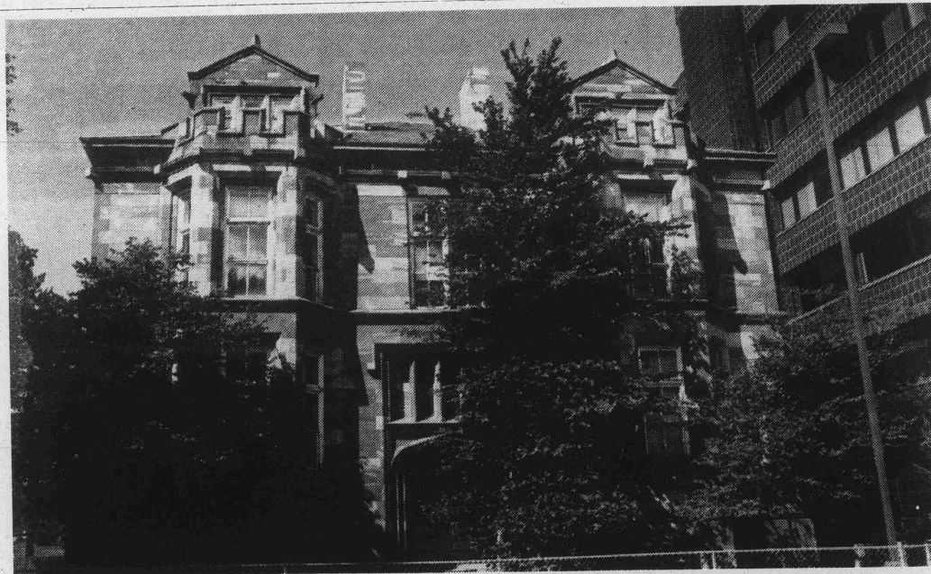
Historic Longyear Hall, which sits in the shadow of the Cohodas Administrative building, may soon be a thing of the past. The NMU Board of Control has already decided to tear down the building. (Paul Brown photo)
