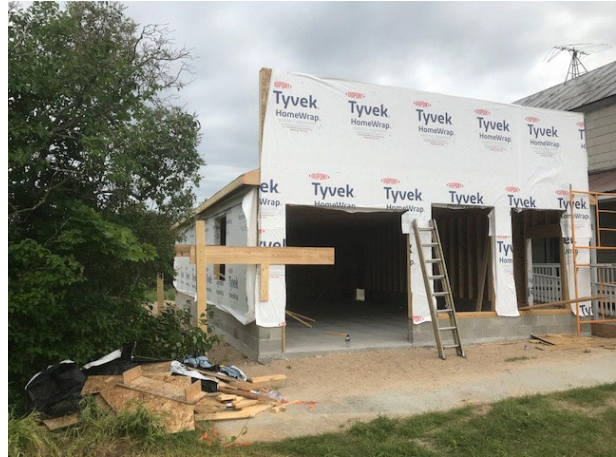
Building the new garage 2020. Thank you RAM construction.
