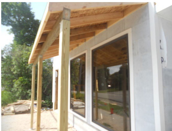
Front of garage with exhibit room 2021.
