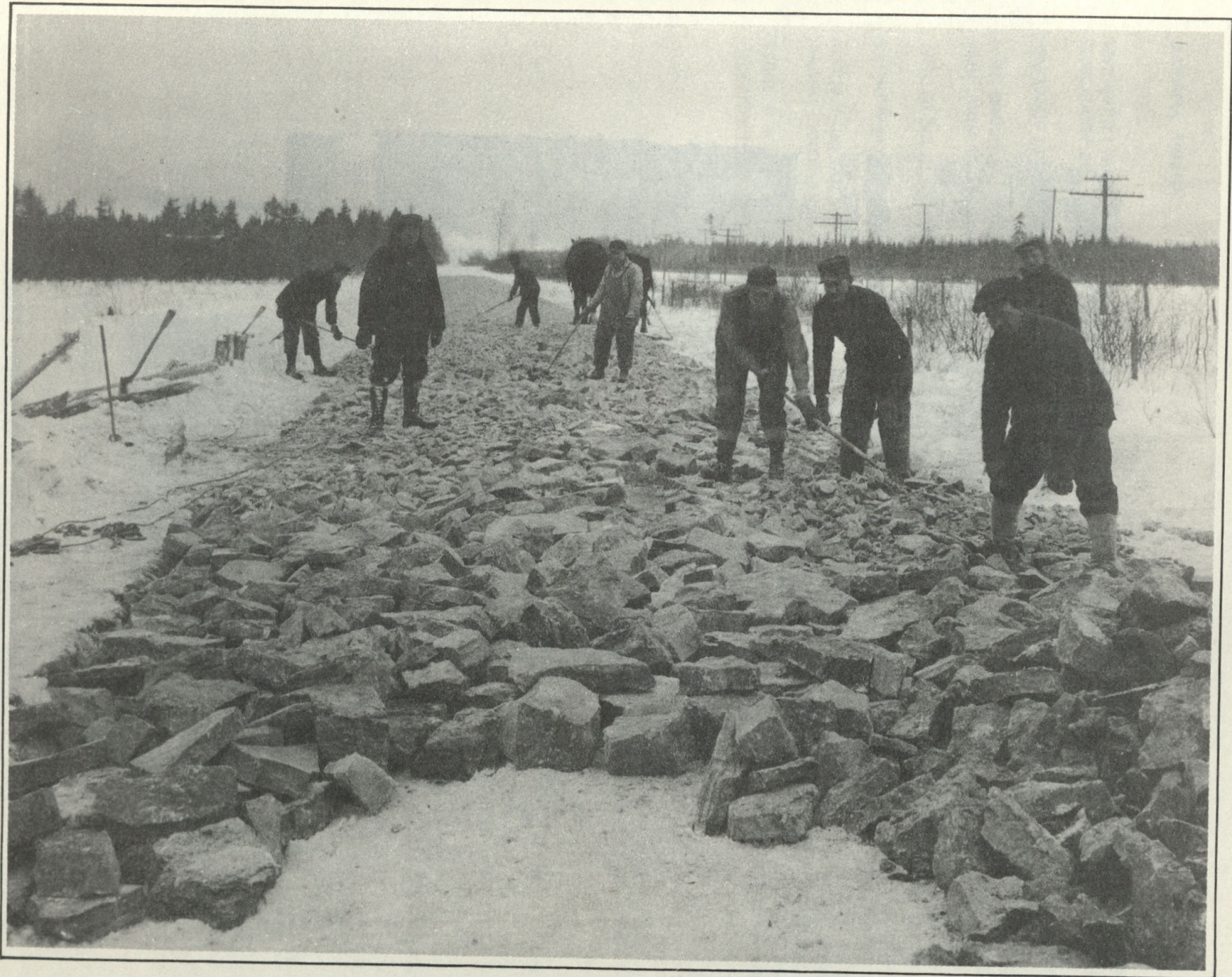
WPA Road Crew working in the National Mine Area
