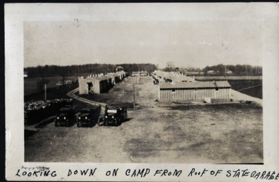
LOOKING DOWN ON CAMP FROM RUF OF STEEL GARAGE
