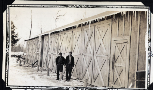
Belle Project - Conservation Garage
