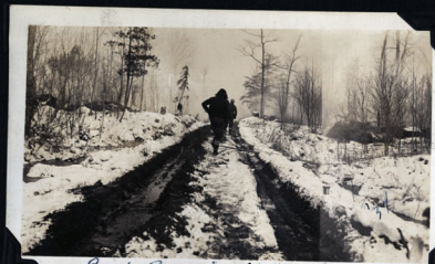
Road Repairing (Mud Hogs)
