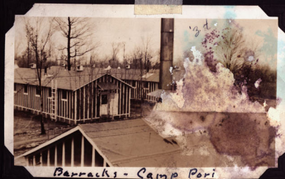
Barracks - Camp Pori
