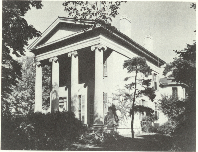
The Wilson-Wahr House, 126 N. Division Street, is one of twelve structures preserved in Ann Arbor's Division Street Historic District. Courtesy: Bentley Historical Library.
