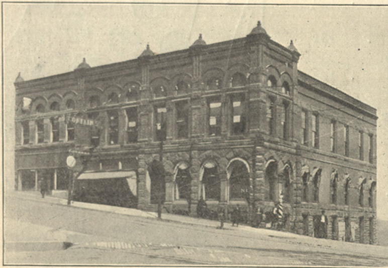
MARQUETTE NATIONAL BANK BUILDING N. E. Corner Front and Washington Streets
