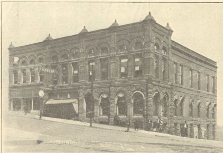
MARQUETTE NATIONAL BANK BUILDING N. E. Corner Front and Washington Streets
