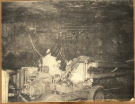
DRILLING A "ROUND" FOR BLASTING
