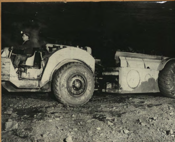
WAGNER ORE TRUCK HAULING 17 TONS OF ROCK
